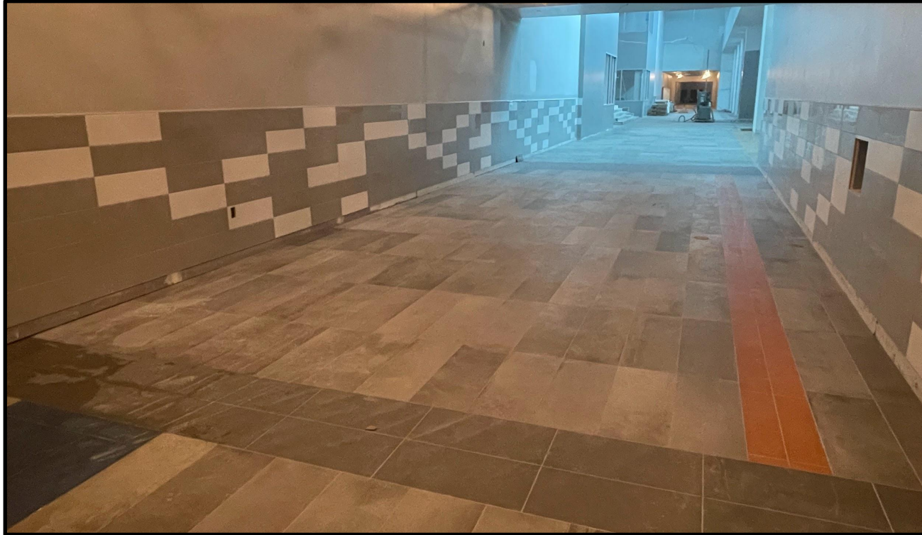
TILE FLOORING AND WAINSCOT
