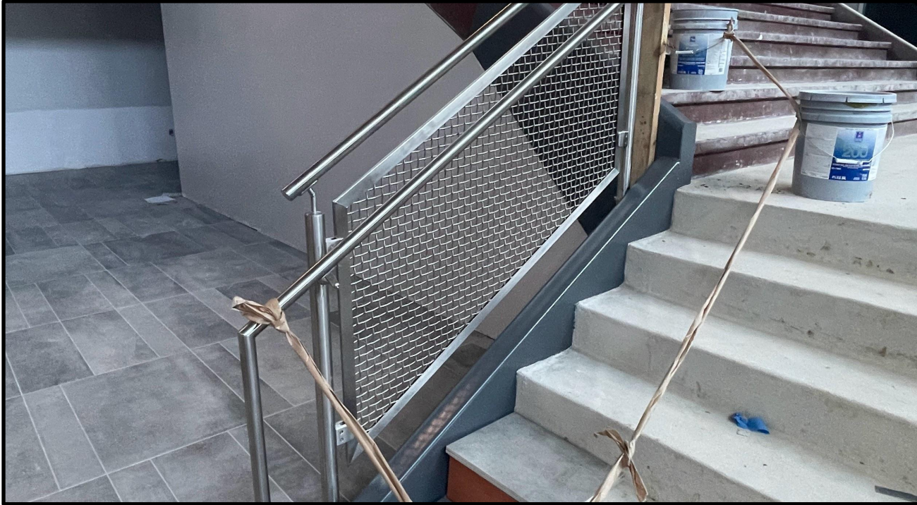
STAIR RAILING MOCK UP
